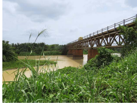
Twifo Faso bridge
