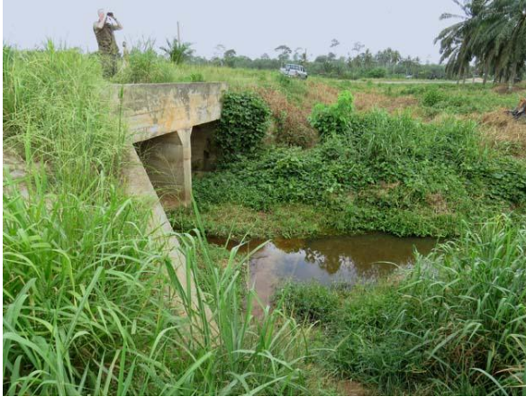
Bridge over Swallow colony
